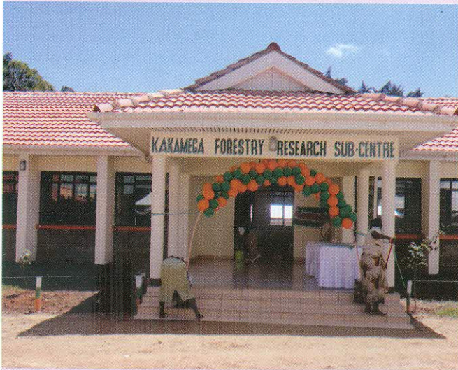
The facade of the new facility at Kakamega.
